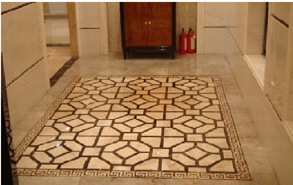
Plate 11. The jointless floor application with laminated marble plates
