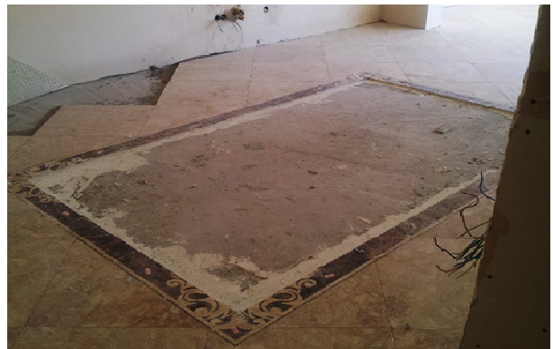
Plate 7. Application of the laminated marble plates
