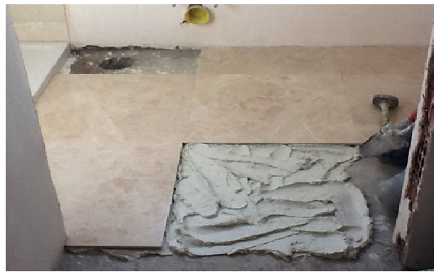
Plate 8. Application of the marble plates
