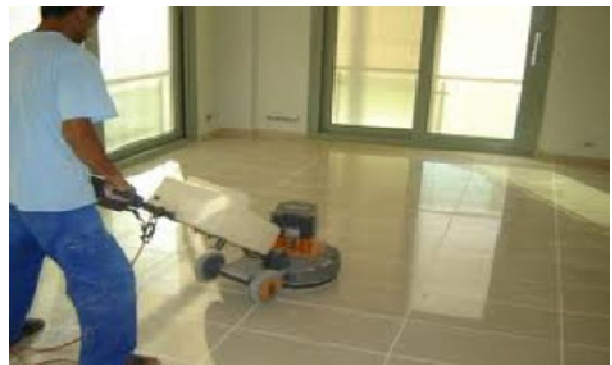
Plate 14. Cleaning and polishing process of the marble floor (Source: Faroz Group, 2015)
