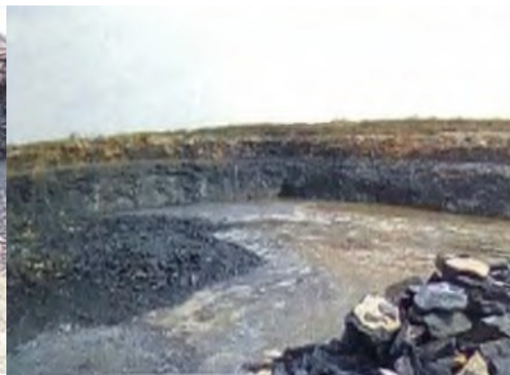
B. Stormwater accumulation at mine-pit
