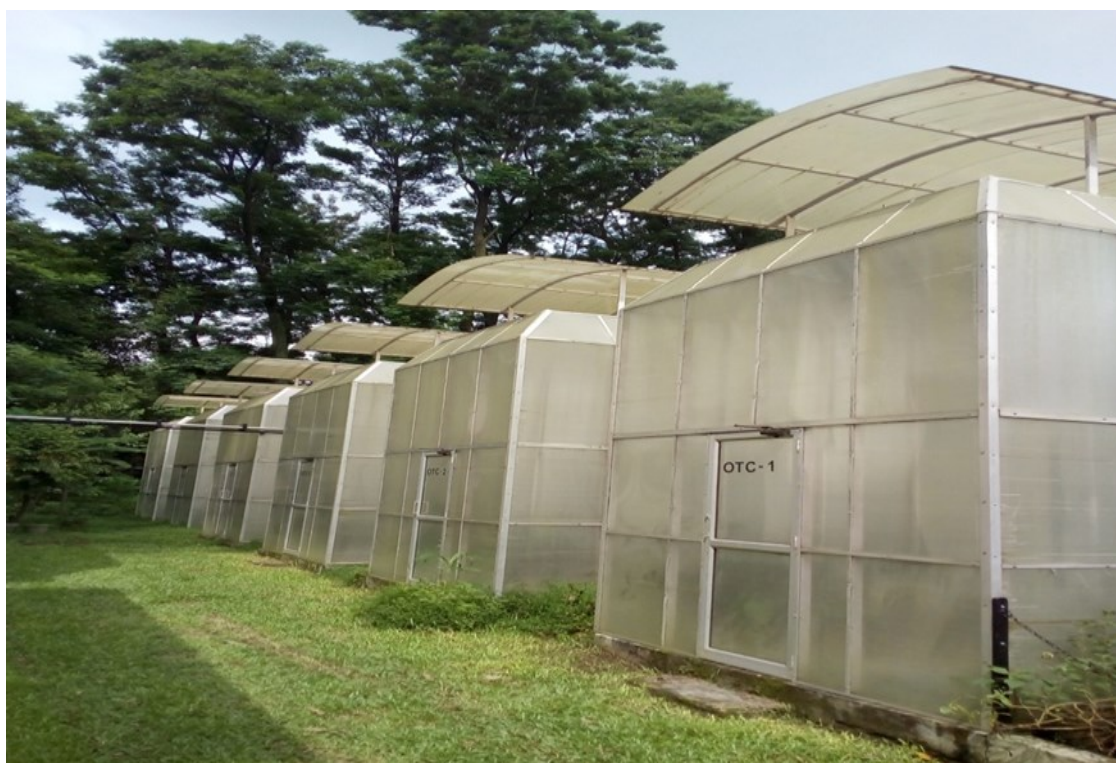
Fig.1. Open Top Chamber Facility in Forest Research Institute, Dehradun
