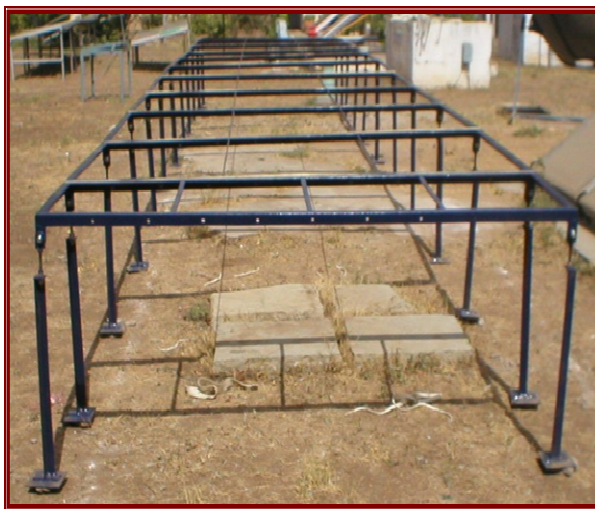
Fig. 1. Dryer supporting structure.
